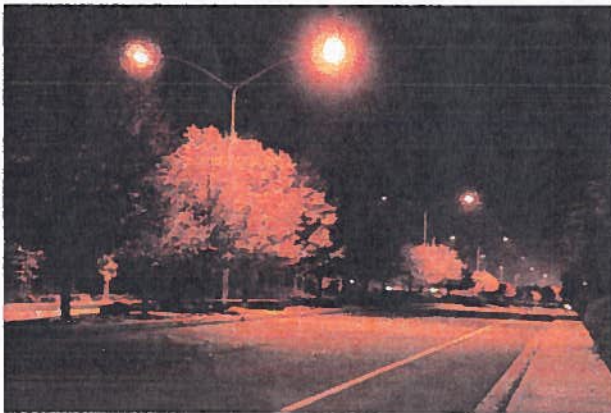
Figure 1: HPS lighting on Las Positas Road in Livermore
